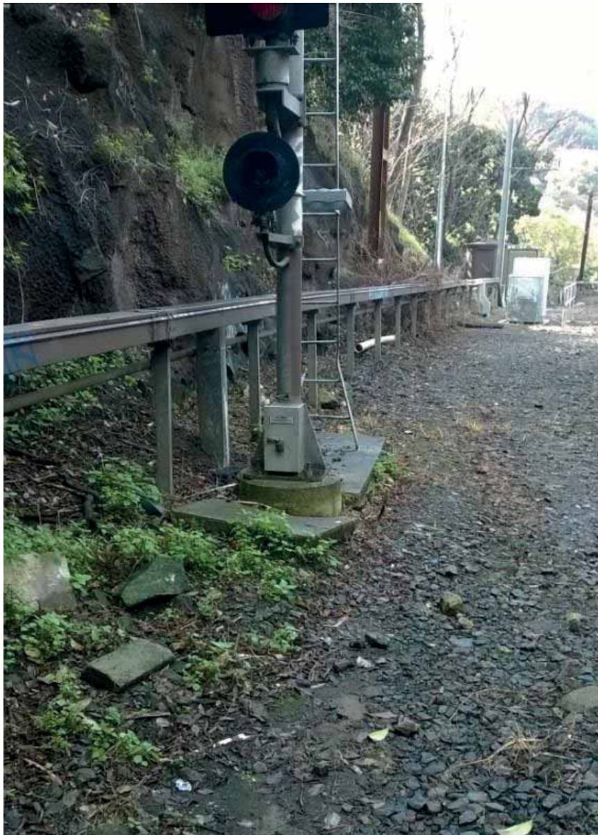
Signal NS 298 CS to be moved to new location due to path alignment conflict however creates a signal sighting issue, rock bolting and repeater signal required.
