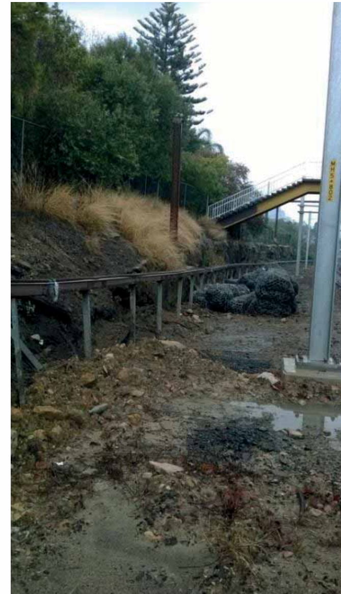
View to Lavender Bay - Cut and groom works required to allow path and lighting. GST to be relocated behind new fence (adjacent to structure).
