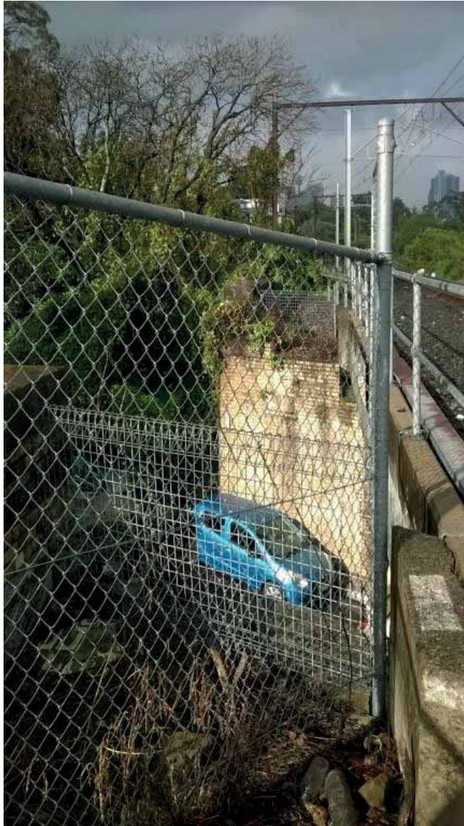
View of abutment area of Waverton side pedestrian walkway. Retaining wall structure required (Wing wall) to enable path and lighting.
