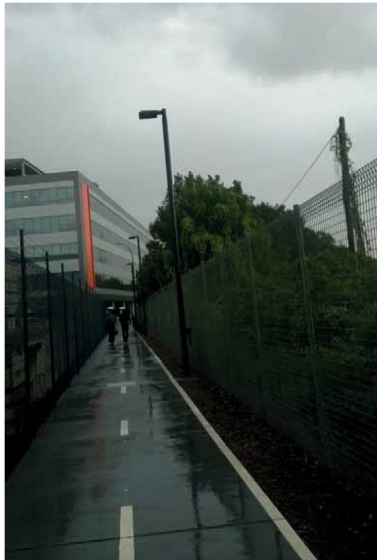
Lighting example used for pricing (unless specified otherwise) - Shows (proposed) lighting and lighting spacing (approx 25 mtrs).
