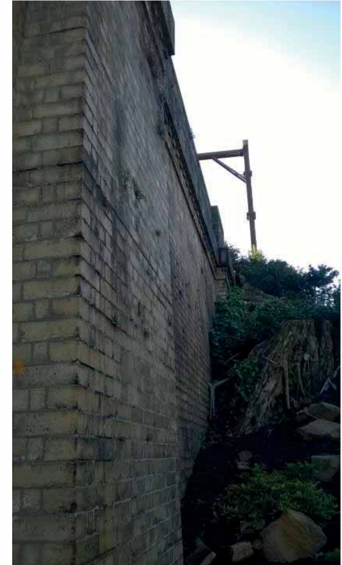
Wing wall to a transition retaining wall (approx. 30 mtrs) structure required to allow adequate path and lighting.
