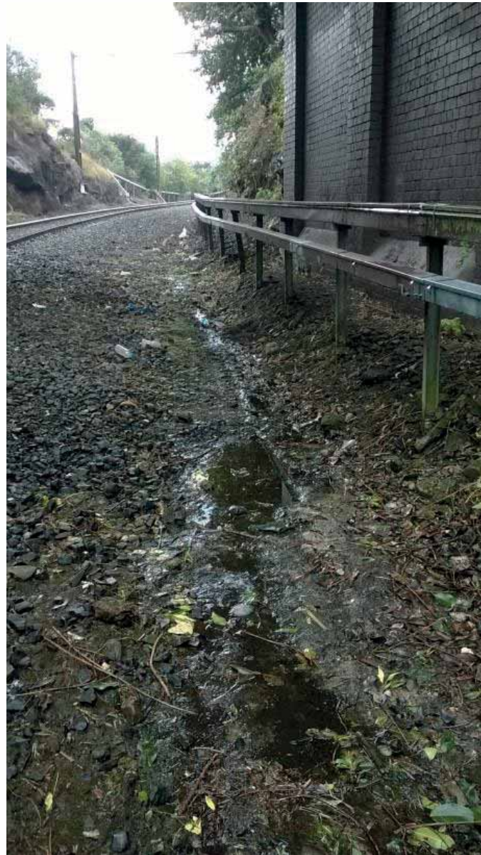
Existing surface water at Victoria St OB. Assume path subgrade to be built up to facilitate drainage to new track drainage. GST relocation.
