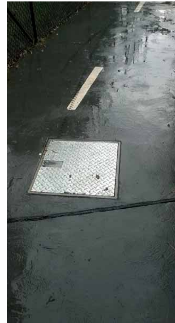
Close up of proposed lighting conduit pit in path and pit lid detail.
