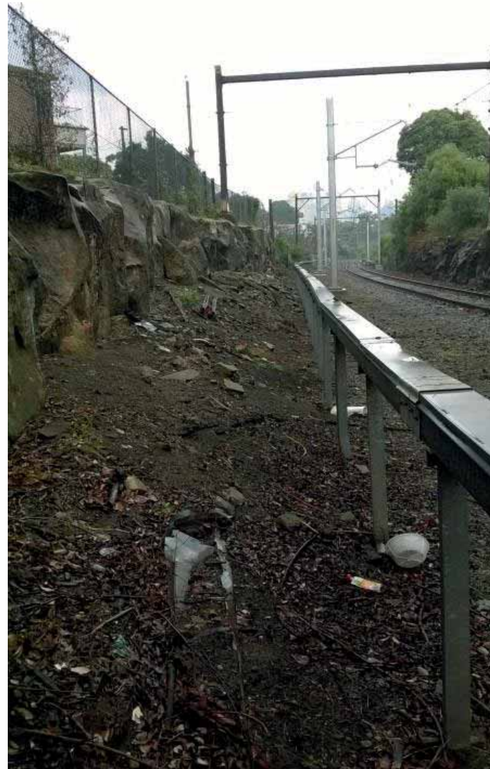
Cut and groom required to allow for adequate width for path and lighting. Assume rock bolt allowance to stabilise rock cutting.
