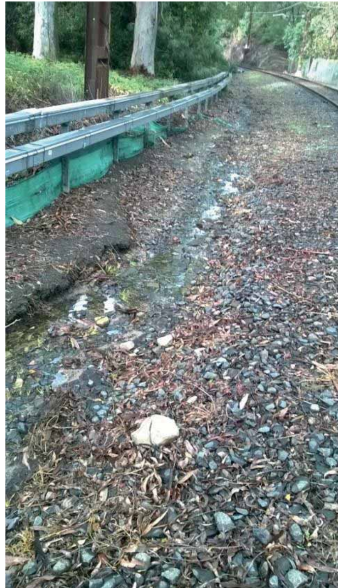
Munro St. Standing water and erosion. GST to be moved behind proposed fence. Vegetation to be cleared new erosion protection and boundary fence required (adjacent property owners) Path on built up subgrade to facilitate run off to new track drainage.
