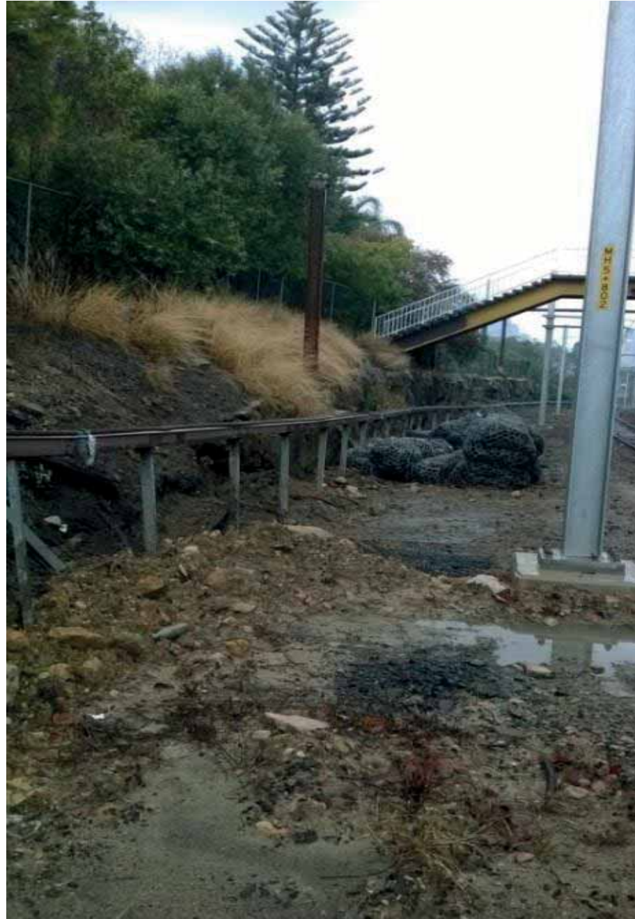
Cut and groom required to allow for adequate width for path and lighting. Assume rock bolt allowance to stabilise rock cutting.
