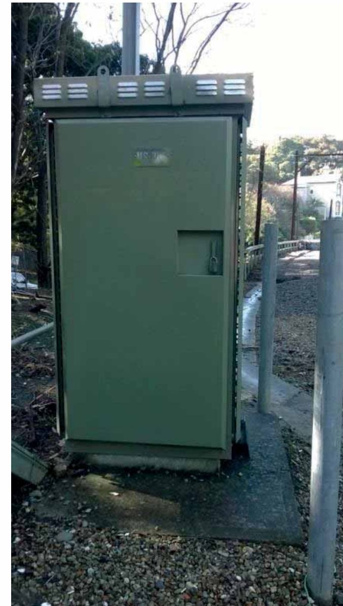
Signal cabinet NS 298 CS to be moved to new location due to path alignment conflict.
