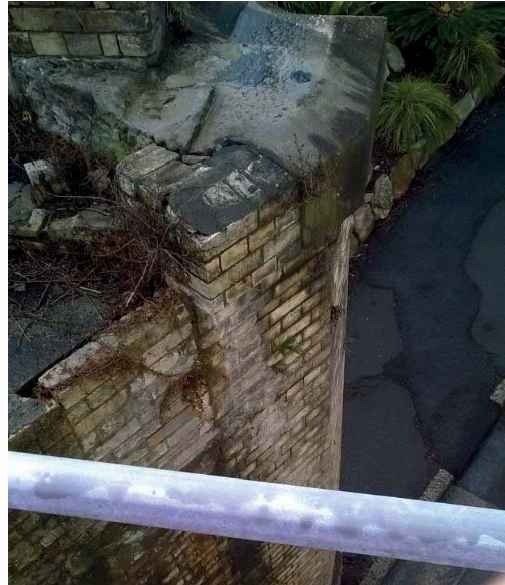
Existing abutment wing wall repair and strengthening required.
